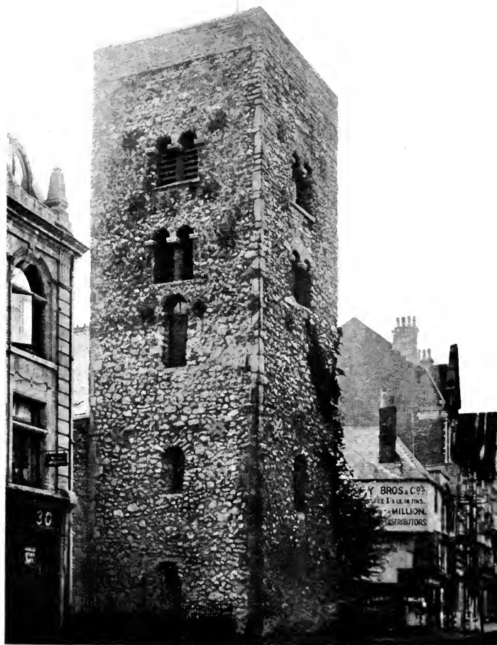
FIG. 10. S. MICHAEL'S TOWER (c. 1071)
